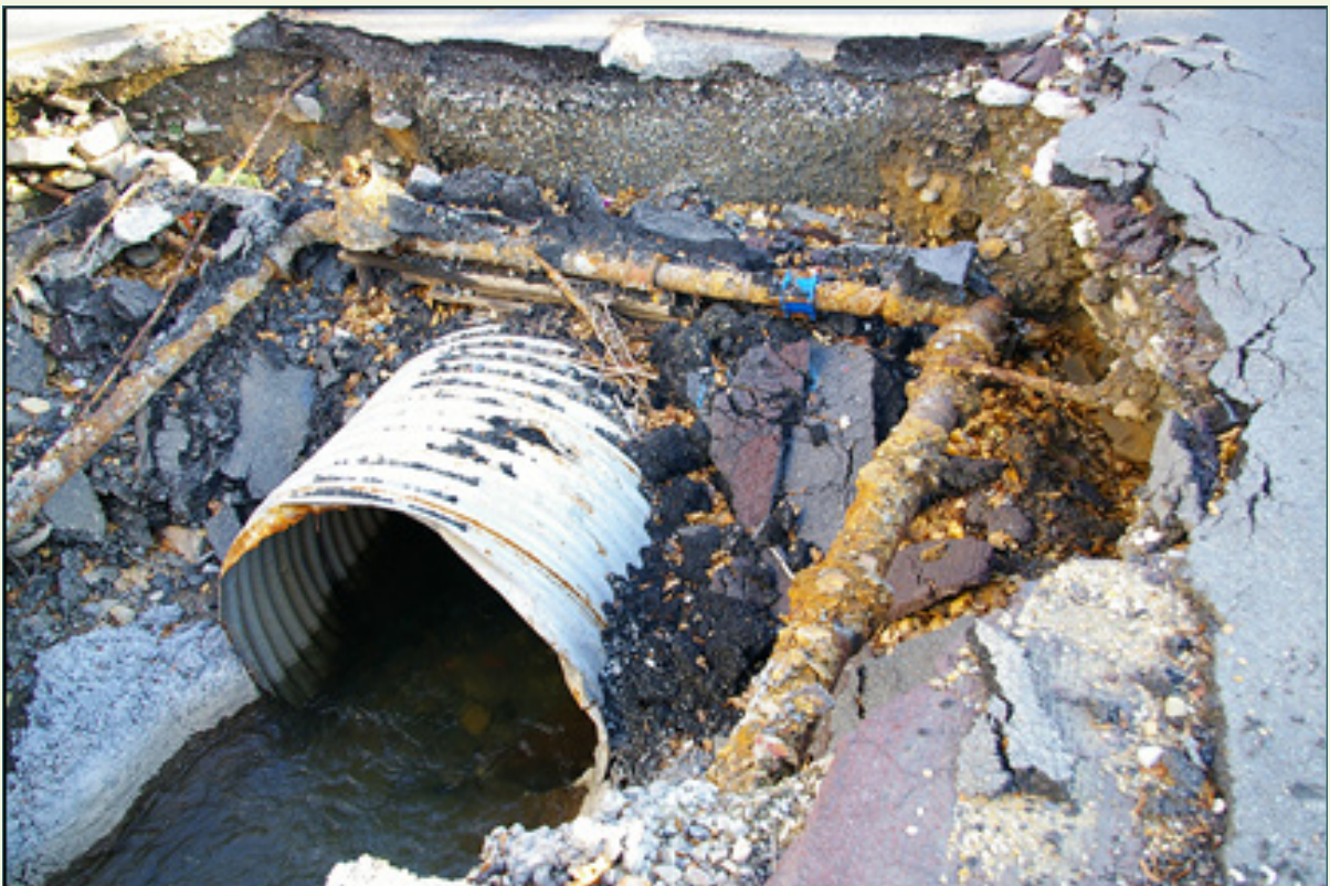
Figure 2. Linking the activities of maintenance crews with the asset management program can be important to asset management success.
