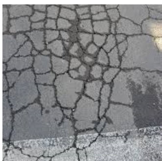
Alligator Cracking
