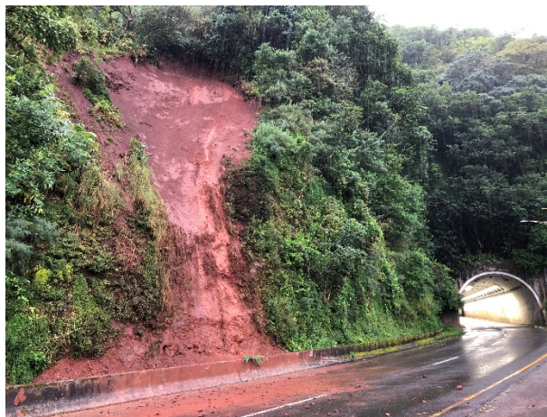
Bulk of the debris is removed at the landslide location at the Kailua bound direction. The slope along the Honolulu bound direction needs to be stabilized before it can be reopened.
