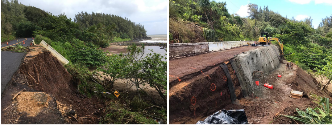
Damage to Kuhio Highway as a result of heavy rains in April 2018. Reconstruction of the roadway with the soil nails occurred from April 2018 to April 2019.
