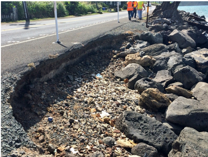
Ocean wave erosion of the pavement and underlying foundation along Kamehameha Highway in Kaaawa
