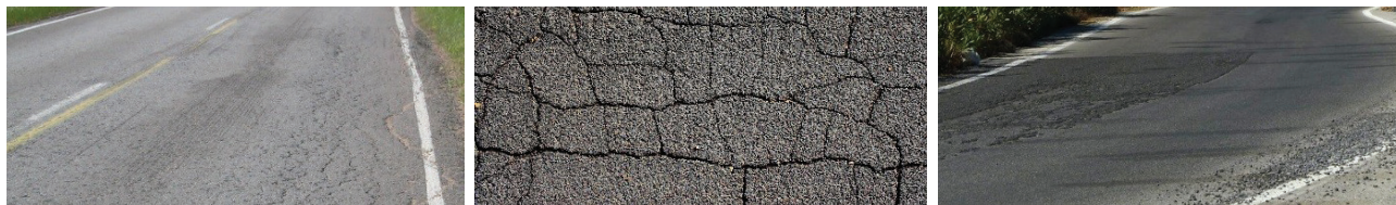
Figure 6 — Examples of Pavement Distress – Rutting, Load Cracking and Raveling (left to right)
