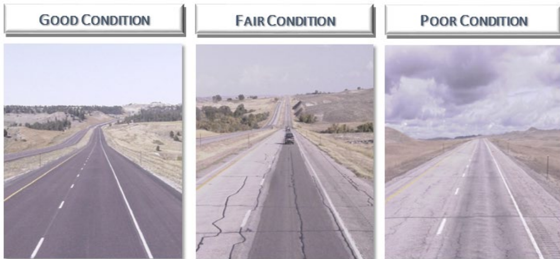
FIGURE 4: VISUAL EXAMPLE OF PAVEMENT CONDITIONS
