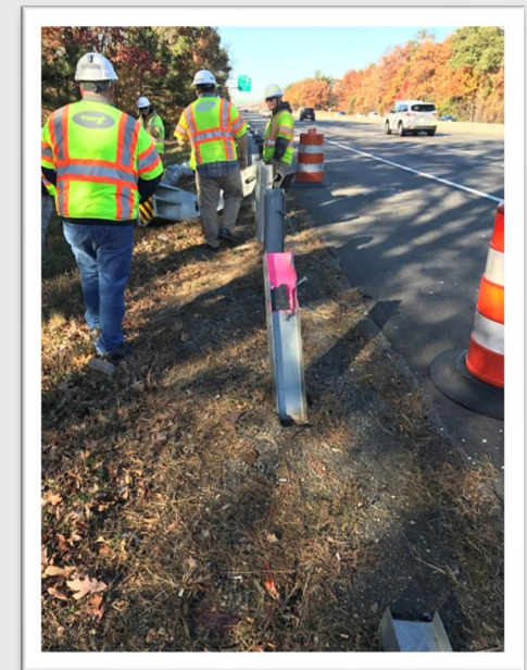
Installing a New Guardrail Asset
