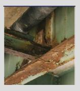
Corroded steel on a bridge girder.
