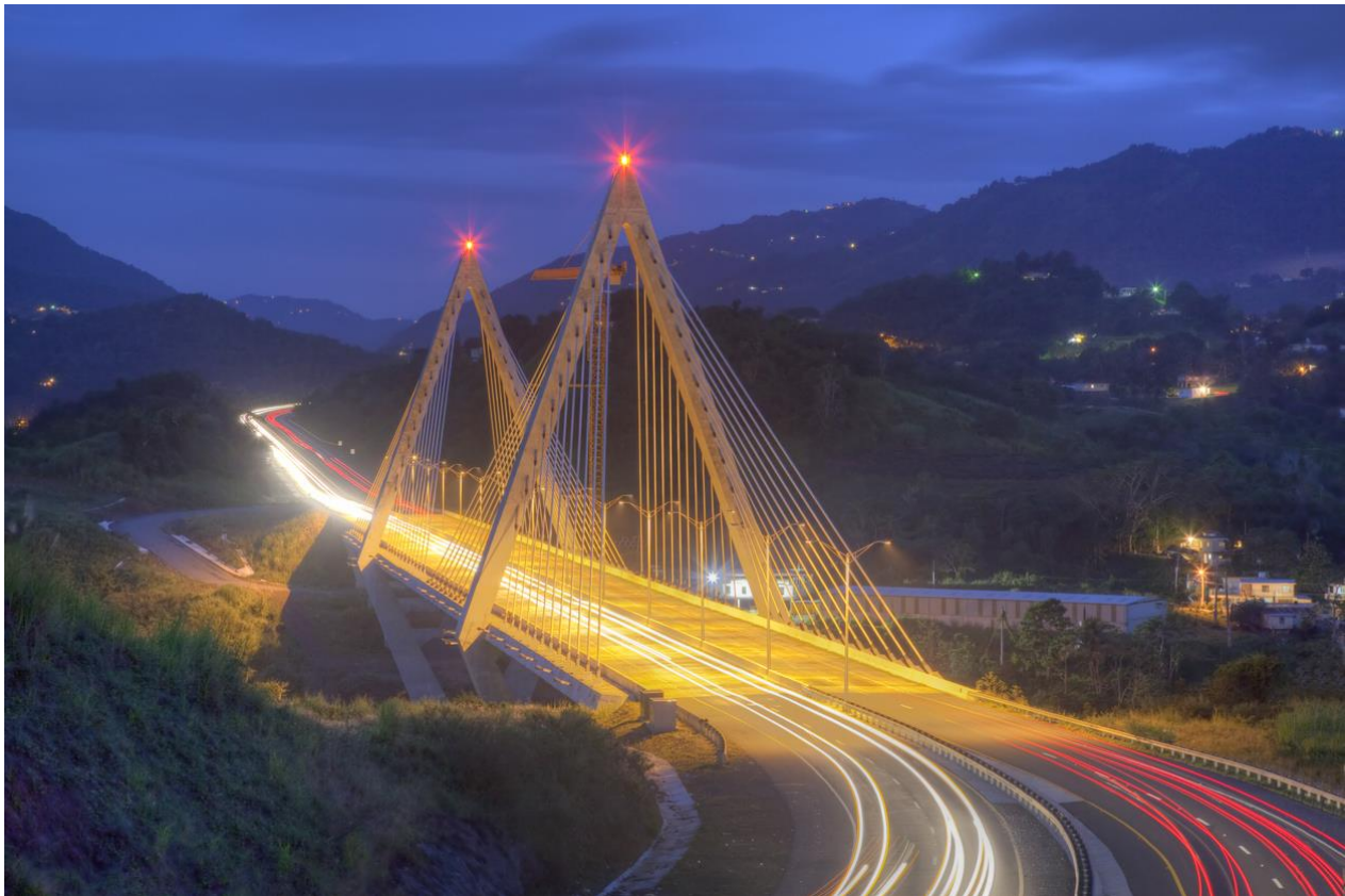
Photo 5-1: Jesús Izcoa Moure Cable-Stayed Bridge connecting Naranjito and Toa Alta
