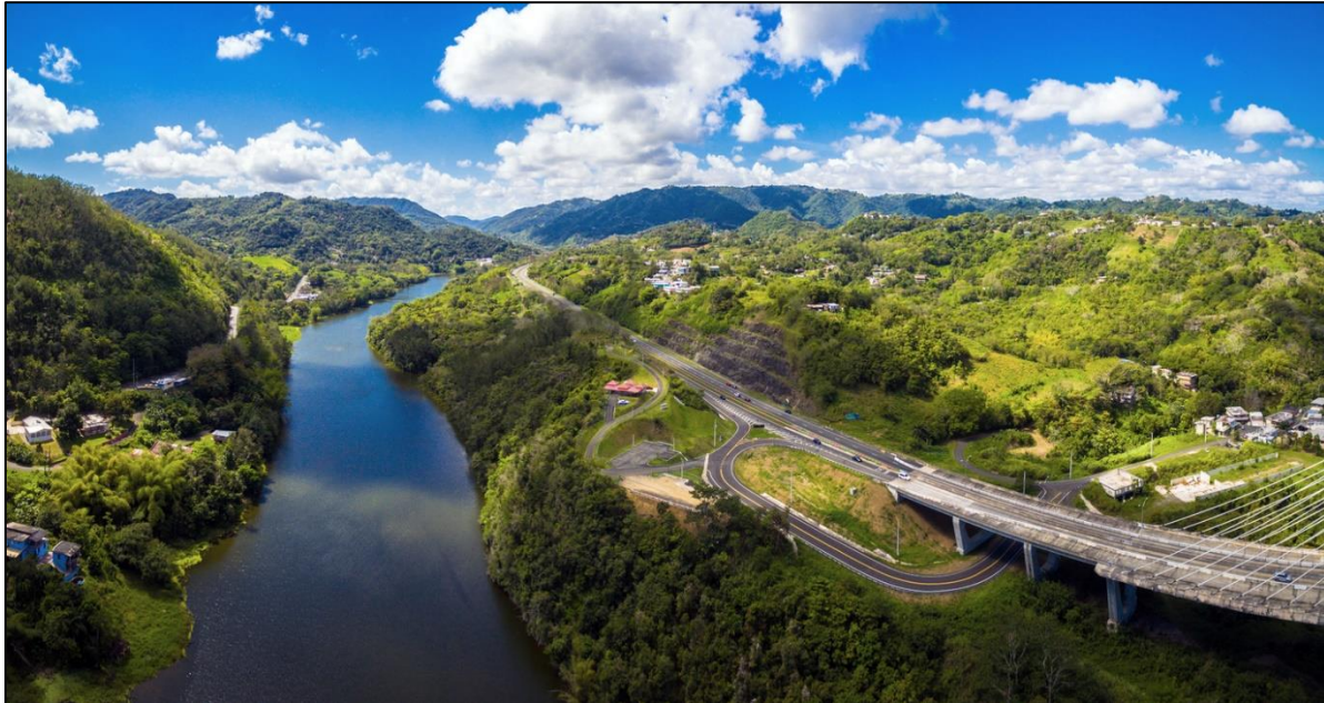
Photo 2-1: La Plata Lake close to Jesús Izcoa Moure Cable-Stayed Bridge
