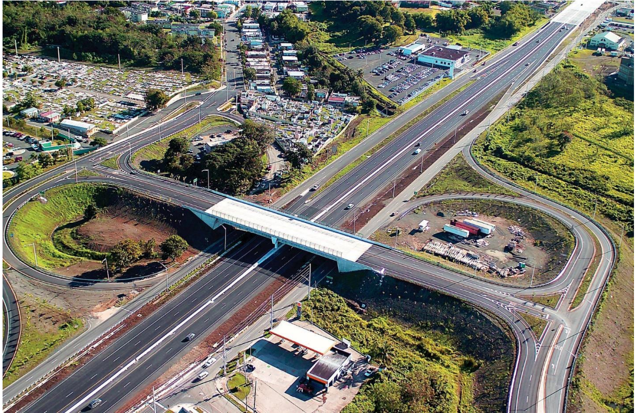
Photo 9-1: PR-2 Expressway Mayagüez - Hormigueros
