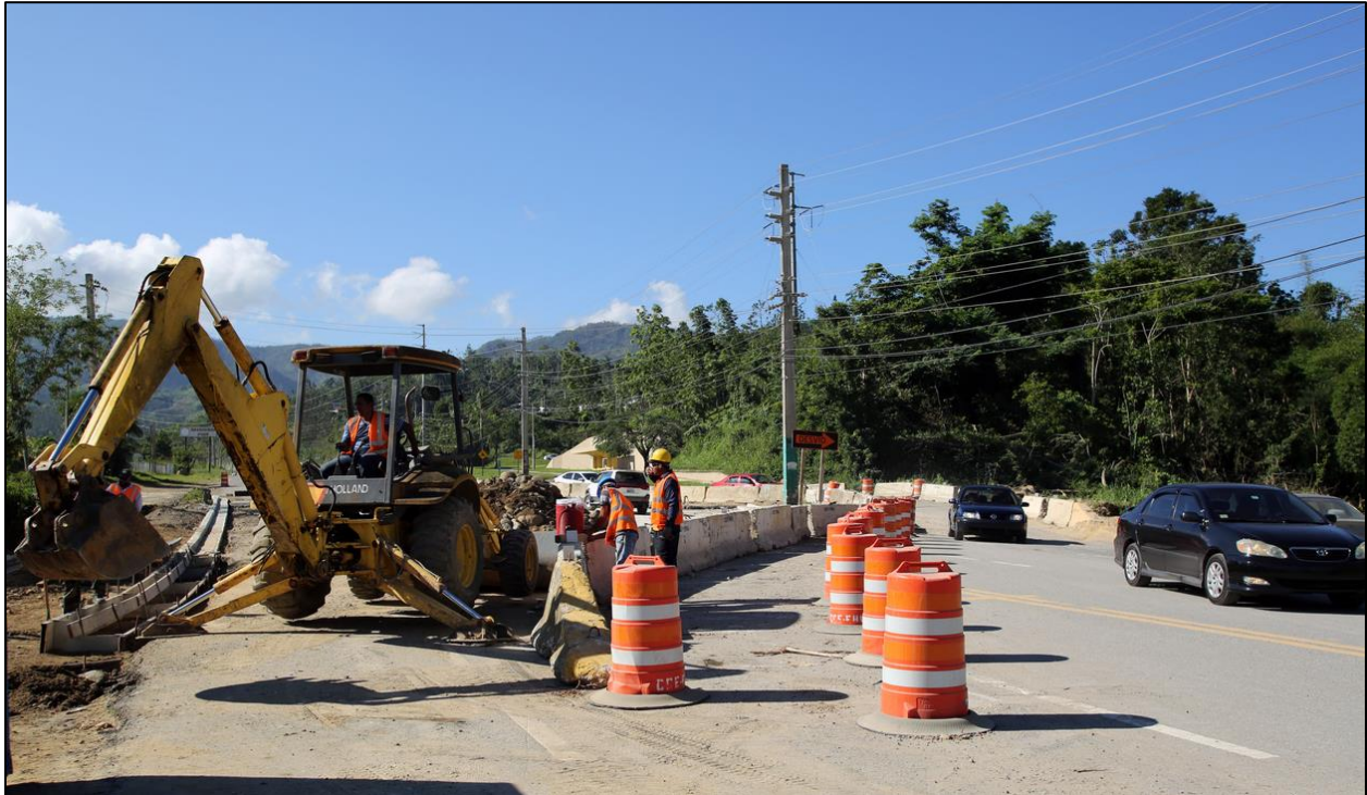
Photo 8-1: Construction to Repair Damage Near Utuado
