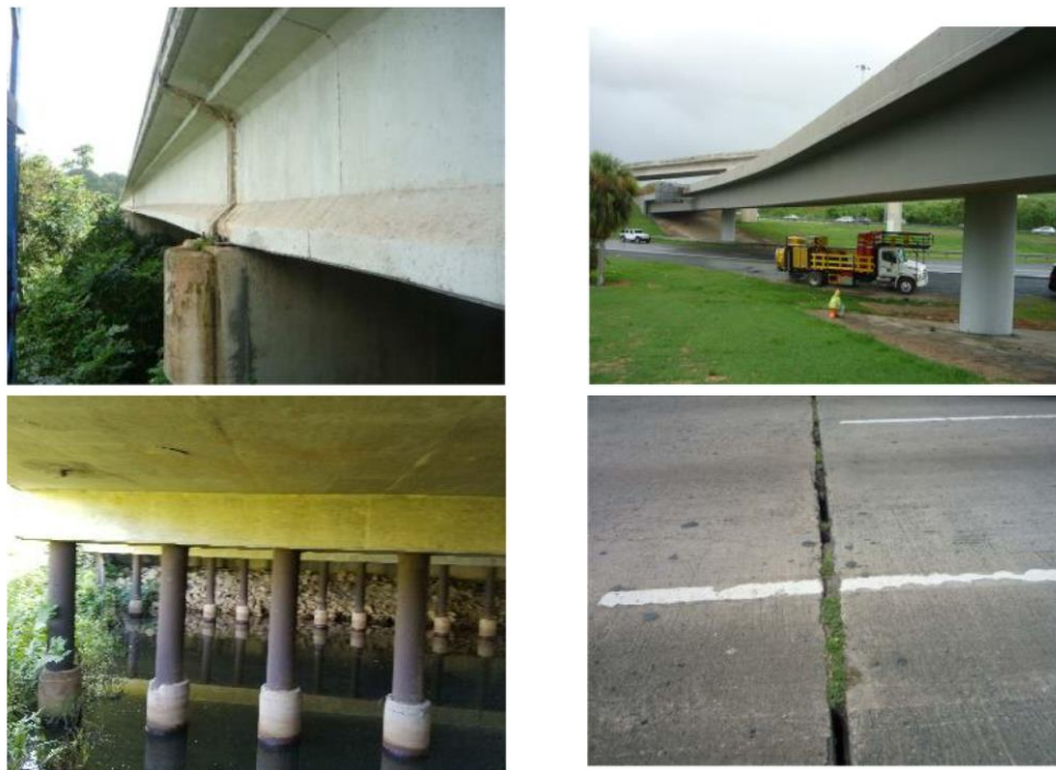
Photo 3-3: Pictures from PRHTA Bridge Inspections
