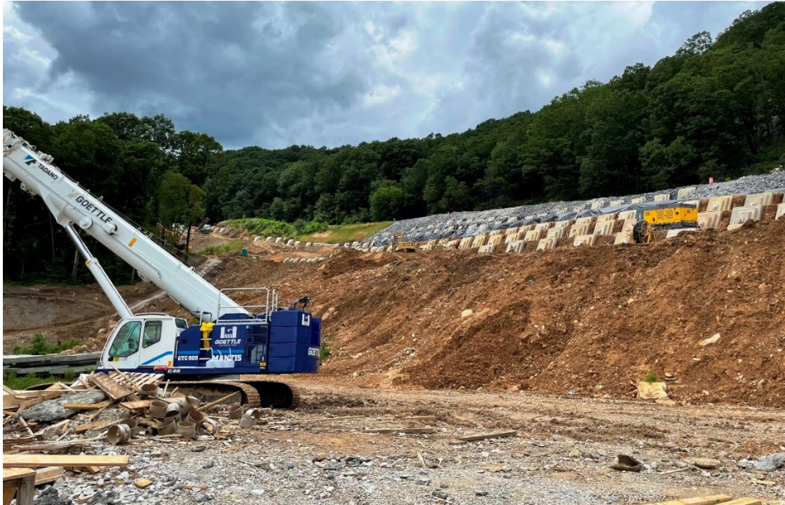
Figure 5-6. Soil nails installed as a landslide stabilization
