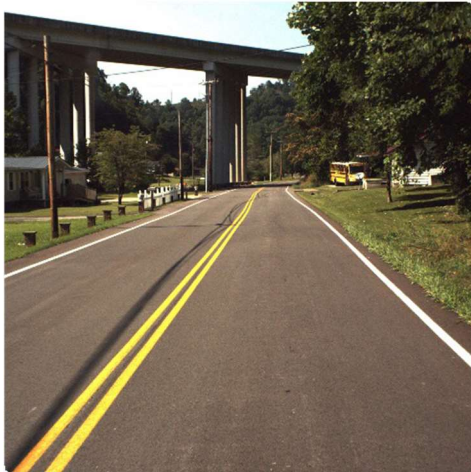
Figure 3-4. Typical MP roadway
