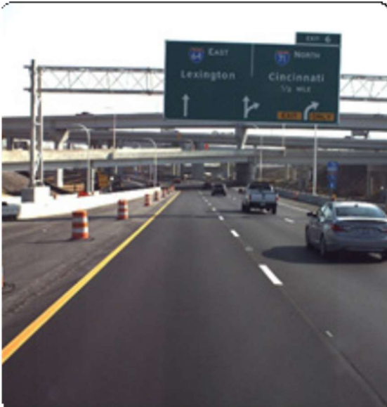
Figure 3-2. Typical interstate roadway
