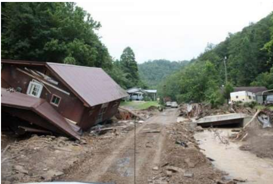
Figure 5- 7. Flood damage in Pike County, KY 2010. Source: Commonwealth of Kentucky Enhanced Hazard Mitigation Plan: 2013 Version.
