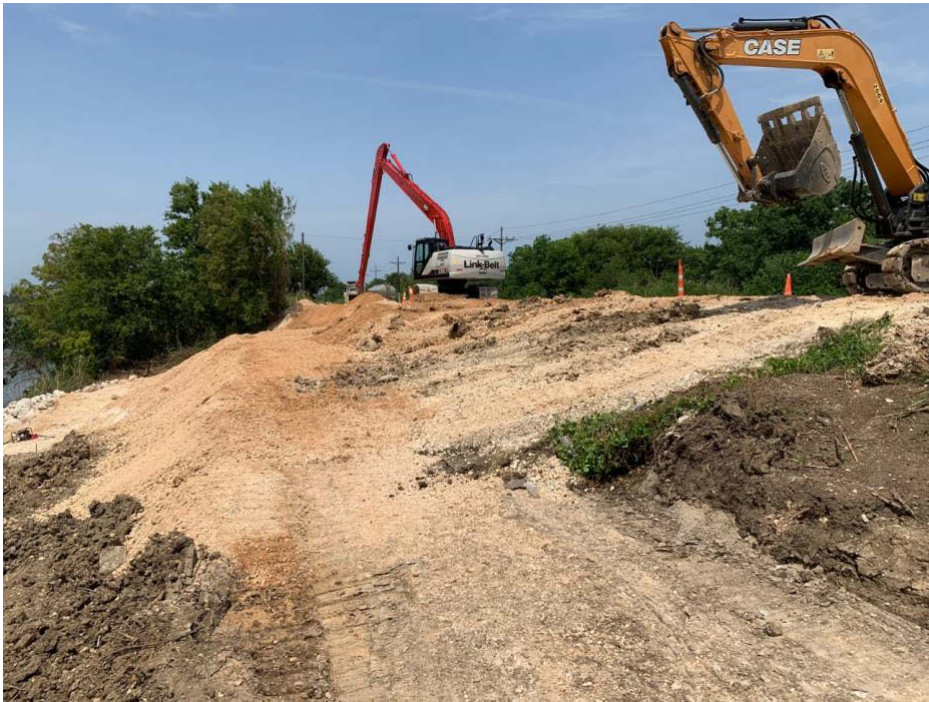
Figure 5-12. State Highway 82 Repairs
