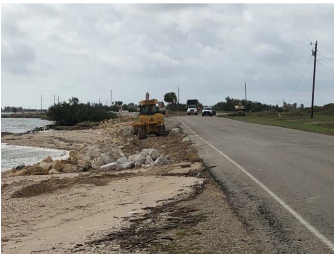
Figure 5-16. State Highway 316 Riprap Placement
