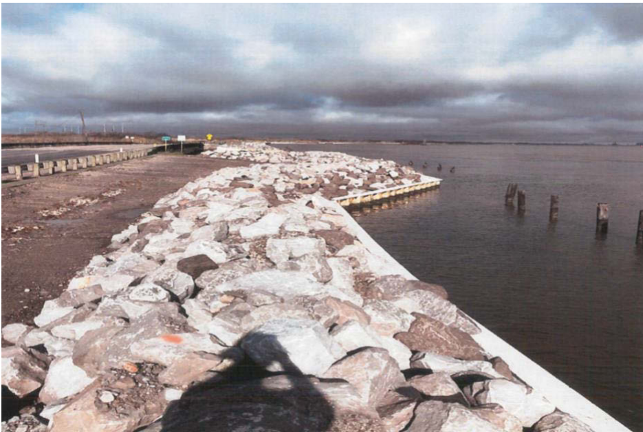
Figure 5-13. State Highway 87 Successful Canal Bank Stabilization
