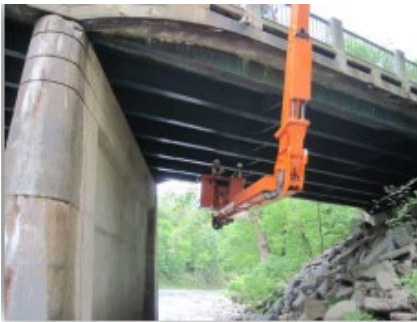
VTrans bridge inspectors at work.
