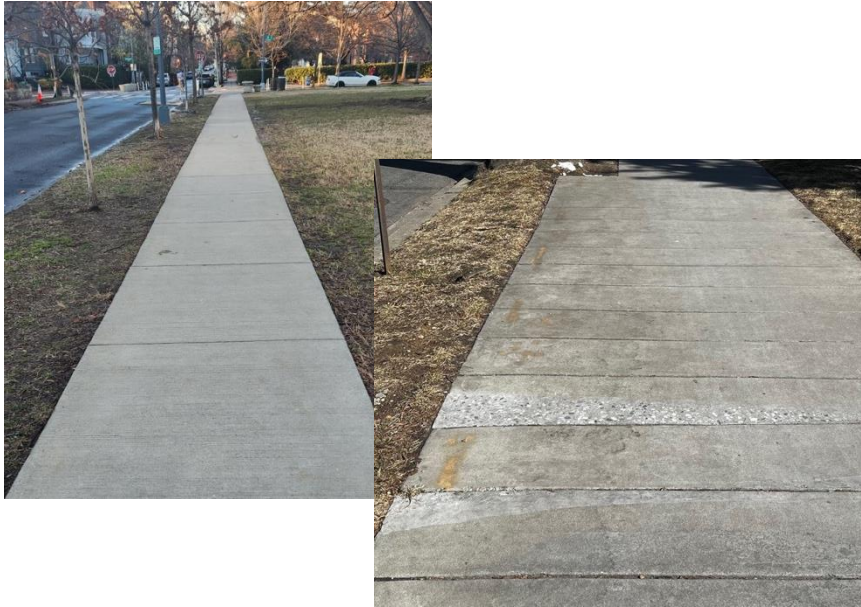
Concrete Sidewalks: horizontal cutting
