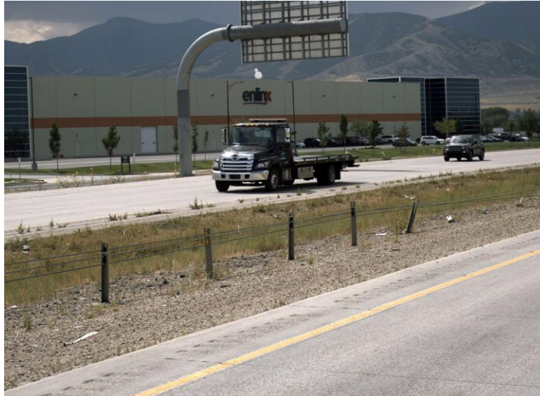
Figure 25. QWEN CASE #4, Image of Broken Cable Barrier Posts along a Road
