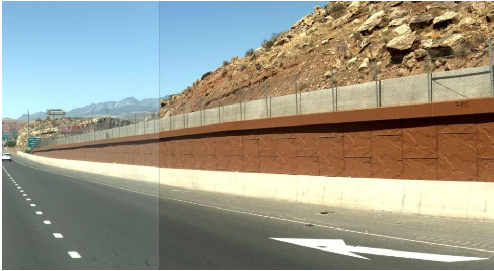
Figure 27. QWEN CASE #6, Image of Highway Retaining Wall
